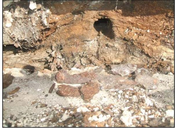
Hole in substantial timber over wheel pit which was fitted with an iron plate, the remains of which are visible
