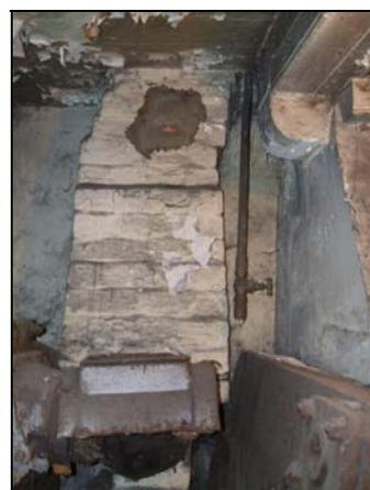
The old coke fired boiler and the chimney which is to be demolished at ground floor level
