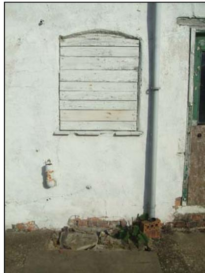
Unknown original feature of the building to be fitted with glazing and a window that was at one time a door
