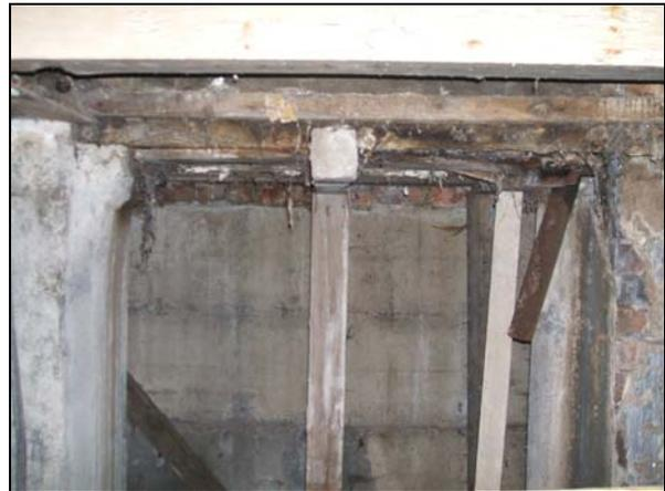
The base of the wheel pit entrance with drainage pipes visible and the shuttering to the top which is to be reopened
