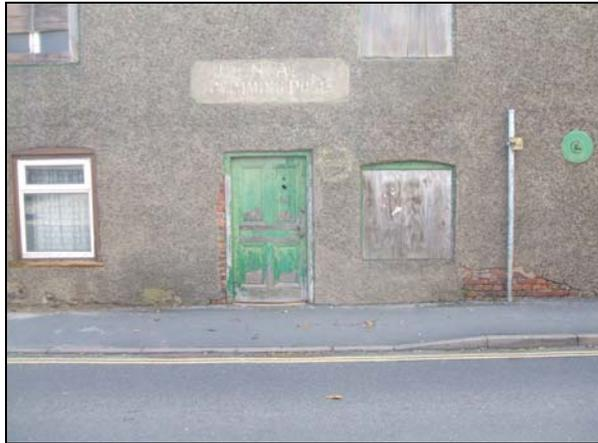
Scarring showing the extent of the lean to extension, the state of the render, front door and an unsympathetic window
