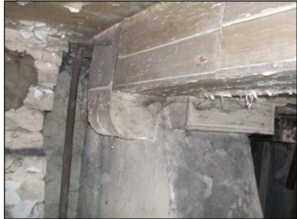
The wheel pit buttress type structure abutting the rear wall and support carrying the load of an existing timber beam
