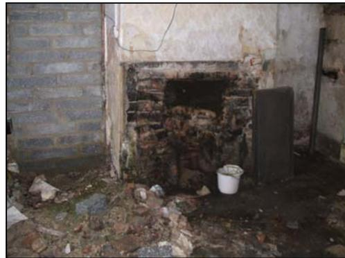
The gable elevation which requires some remedial works and the crumbling chimney breast
