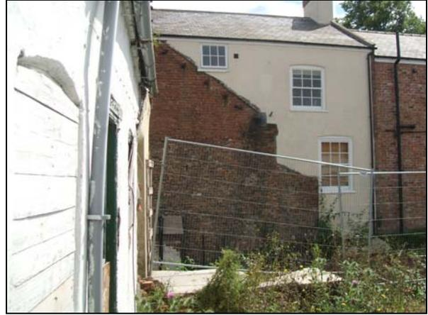
The front elevation and the scarring on No. 38 revealing the extent of the former building at No. 36
