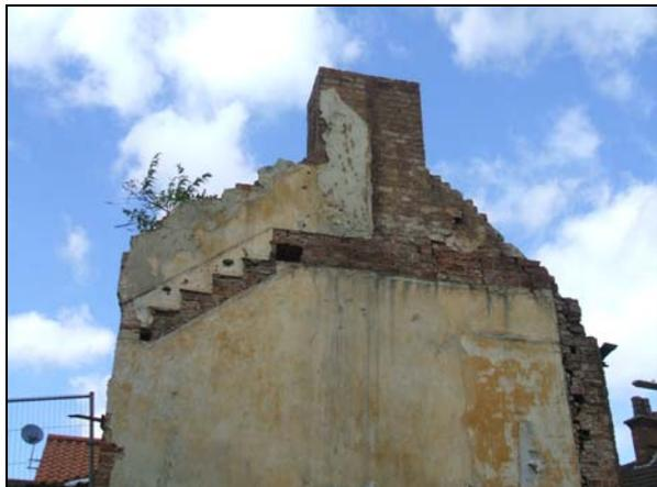
Rear chimney to be reduced in height and side chimney which is to be constructed to its original height
