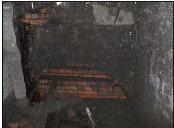
Looking down into the wheel pit and towards the bricked up tailrace within the wheel pit
