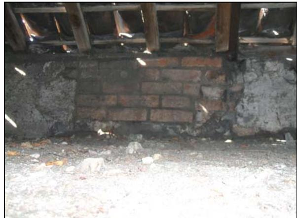
The small timber door originally used to vent the loft space and the bricked up remnants of another (one of at least 5)
