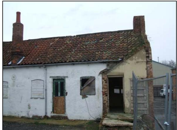
The rear elevation with its boarded up openings and evidence of the demolished extension
