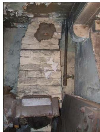
The old coke fired boiler and the chimney which is to be demolished at ground floor level
