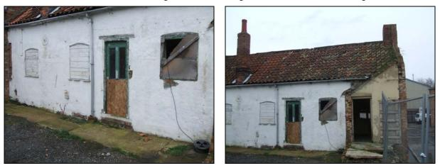
The rear elevation with its boarded up openings and evidence of the demolished extension
