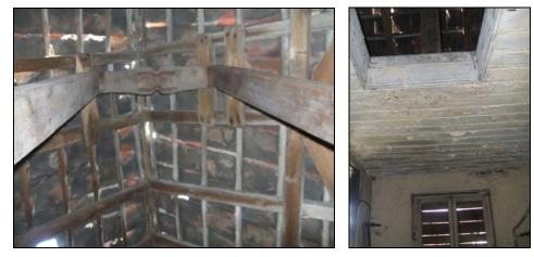
The hoist structure situated over the loft hatch and its relationship with what was originally a doorway at first floor
