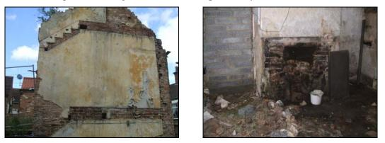
The gable elevation which requires some remedial works and the crumbling chimney breast
