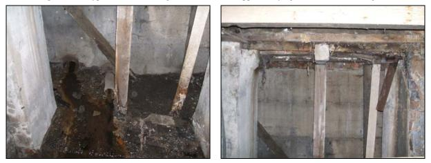
The base of the wheel pit entrance with drainage pipes visible and the shuttering to the top which is to be reopened
