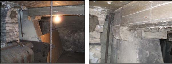
The wheel pit buttress type structure abutting the rear wall and support carrying the load of an existing timber beam
