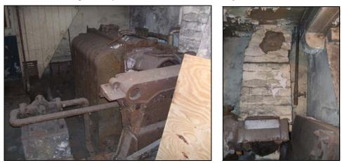
The old coke fired boiler and the chimney which is to be demolished at ground floor level
