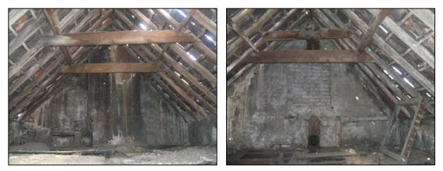
The roof structure looking towards the retained chimney and the blocked up entrance to the former Globe Inn
