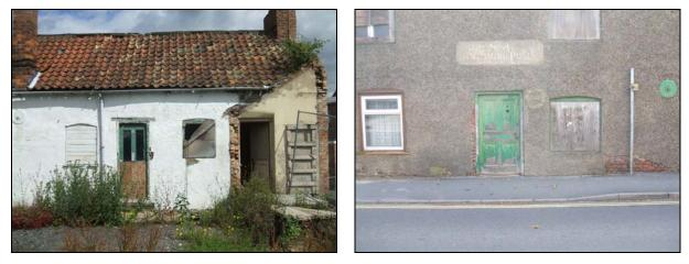
Scarring showing the extent of the lean to extension, the state of the render, front door and an unsympathetic window
