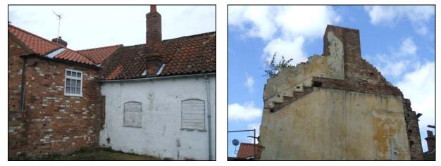
Rear chimney to be reduced in height and side chimney which is to be constructed to its original height
