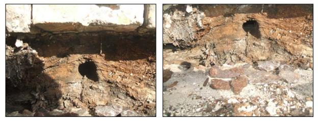
Hole in substantial timber over wheel pit which was fitted with an iron plate, the remains of which are visible
