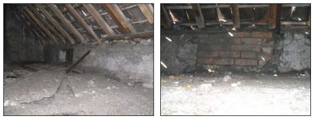
The small timber door originally used to vent the loft space and the bricked up remnants of another (one of at least 5)
