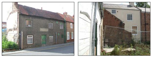
The front elevation and the scarring on No. 38 revealing the extent of the former building at No. 36
