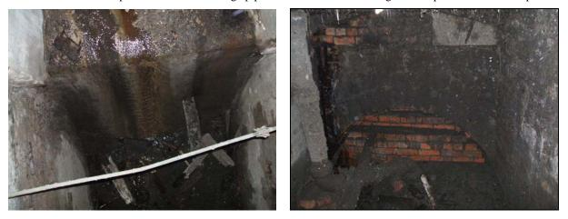
Looking down into the wheel pit and towards the bricked up tailrace within the wheel pit
